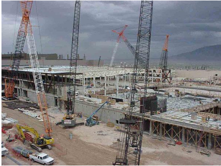
Intel Fab 11x project, Submicron Manufacturing Facility, Rio Rancho, New Mexico: Aug 28, 2000
